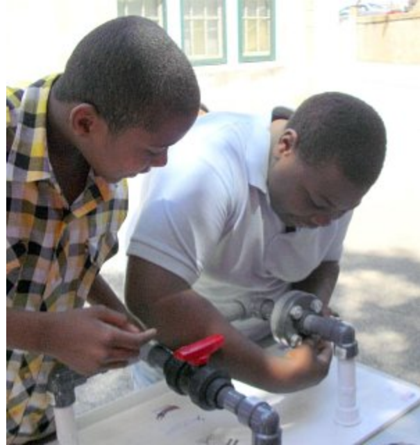
Students from Hoffman Middle School fit pipes during CPS's 5th Quarter.
